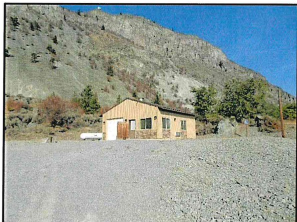
Looking northwest from southwest corner of site
